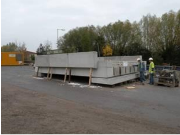
Above: The east side of the 'Laverton Gap' will have the brick pilasters replaced (you can see those on the opposite side) when the bridge is reinstated. The deck beams (below) will be grouted together to form an one integral unit
