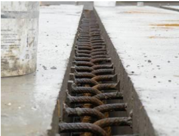
Above: The east side of the 'Laverton Gap' will have the brick pilasters replaced (you can see those on the opposite side) when the bridge is reinstated. The deck beams (below) will be grouted together to form an one integral unit
